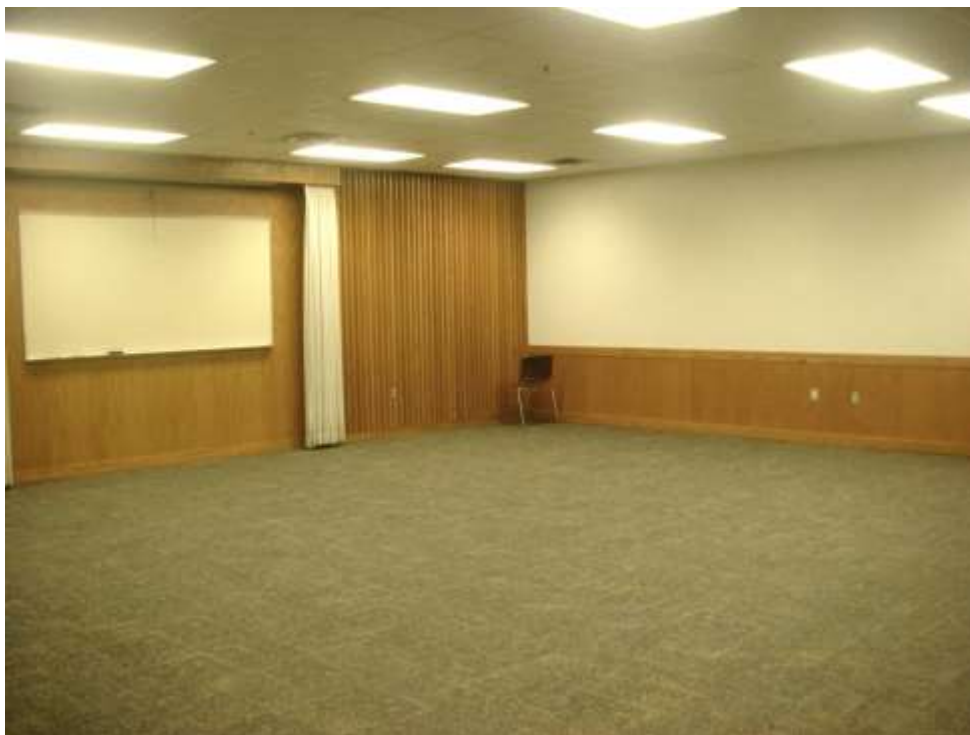
Figure 3.5 A conference room with dimensions 9.3 x 9.2 x 2.7 and volume 231 m 3 . The floor is carpeted cement, the walls are made of wood paneling and drywall, and the ceiling is composed of suspended acoustic tiling.
