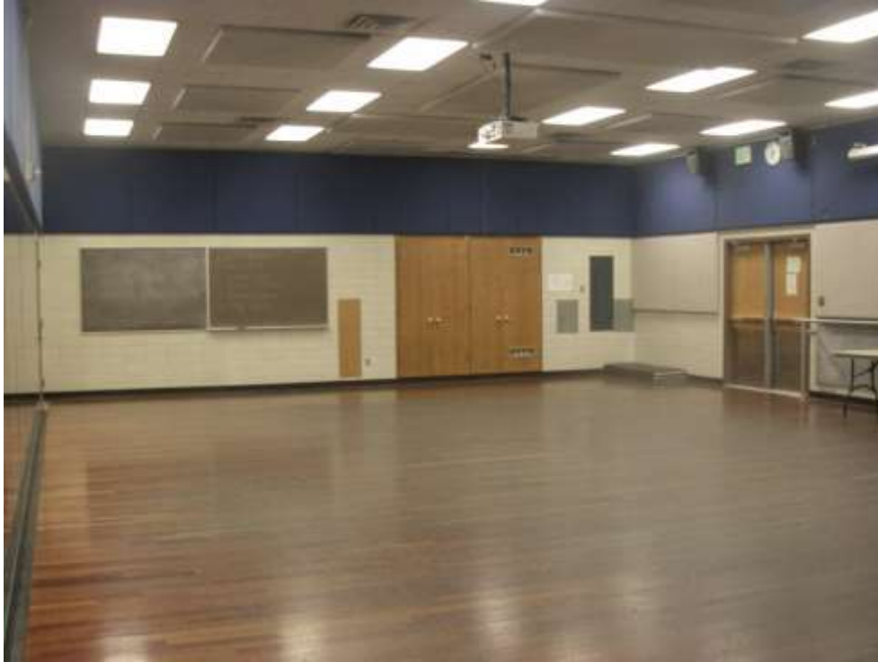
Figure 3.6 A dance studio with dimensions 9.6 x 15.4 x 3.6 m and volume 532 m 3 . The floor is wood, the walls consist of ceramic tile with some absorptive treatment, and the ceiling is composed of acoustic tiling with added absorptive treatments.
